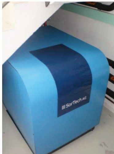
7,5 kW adsorption chiller used in Perpignan
