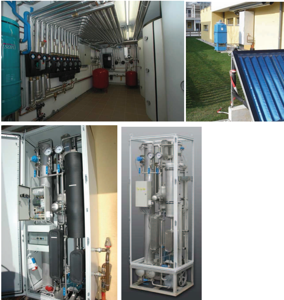
Figure 3: View of the utility room [upper left, Bachler], the outside situation with the wet cooling tower and the absorption machine [upper right, Bachler] and the inside of the cooling machine [lower left / right, Pink]
